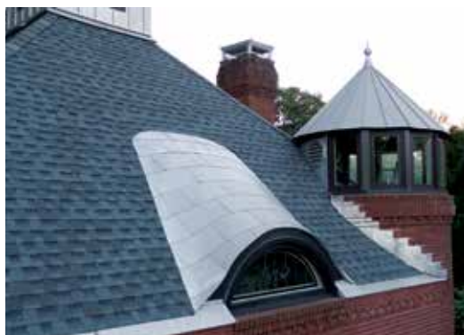
Architect's Residence, Andover, MA
